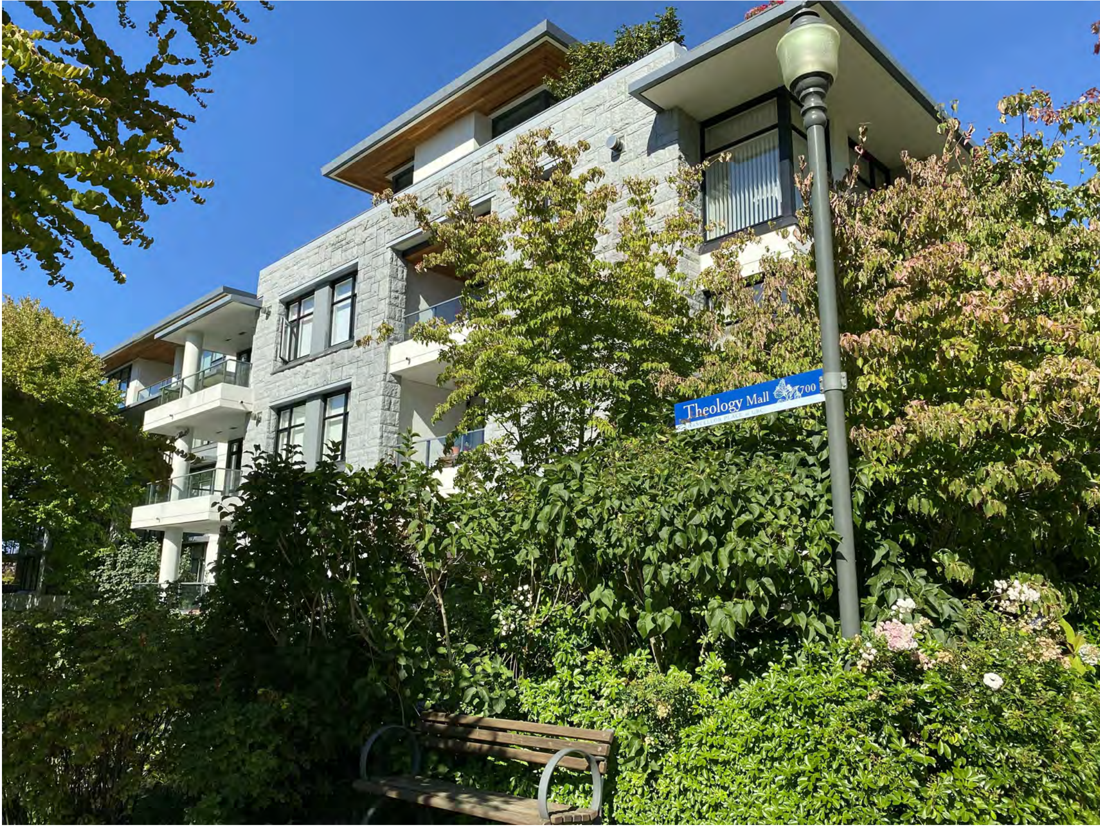
Fig. 5 - 5958 Iona Dr- Typical (Grey) Accent Colour, Quarried Stone, and "Slate Grey" Concrete Slab Edges w/ "White" painted Concrete Soffits, and "Wood-tone Soffits"
