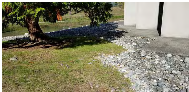
View G13 Sheet L5 (G13:L5) existing site conditions | roots of cedar visible in foreground of photo - meters outside of tree dripline | critical root zone in conflict with required seismic upgrade excavation
