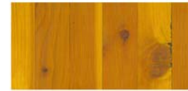
1. Wood Structure & Soffits
