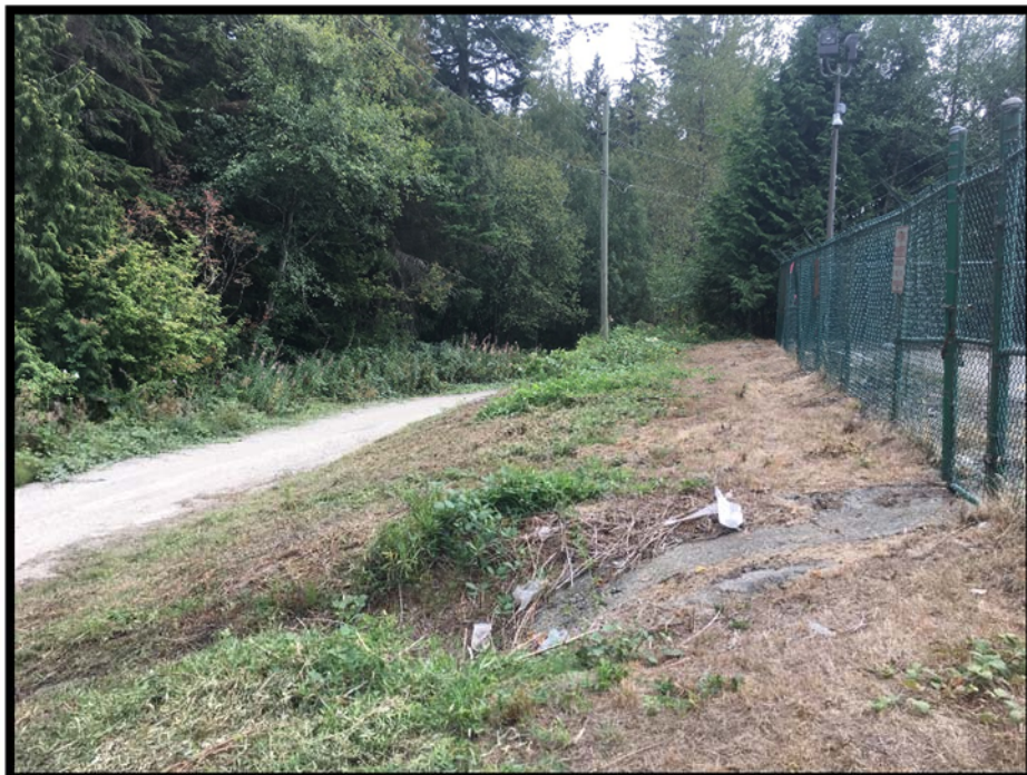
Photograph 4: A slope near the roadway at the eastern portion of the Site, which indicates that fill materials have been brought onto the Site.
