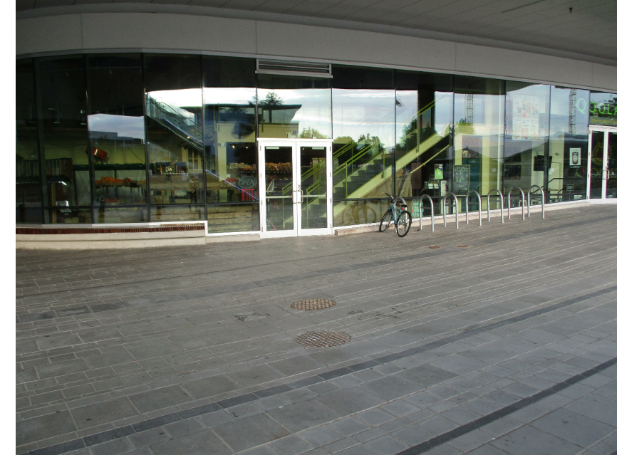
4-CRU'S @ AMS BUILDING
